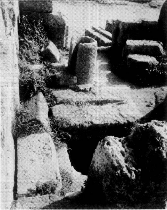
Figure 22.15. Water channel at Selinus, covered with stone slabs. A wellhead gives access to the flowing water below. Compare with Fig. 16.15, a very similar arrangement at Athens. The channel held runoff water which could be re-used to water animals, for crafts manufacturing in domestic courtyards or shops, and to water down the streets for evaporative cooling.
