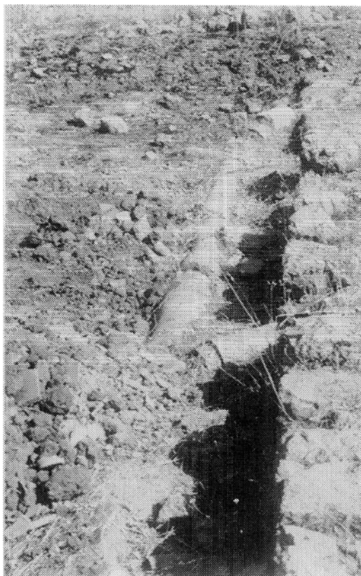
Figure 16.3. Pipes with V-joint, supplying the "Bath of Aphrodite" near Papa Hill in Morgantina. V-joints are known in pipelines of the Athenian Agora also. Each pipe is about .66 m long.
