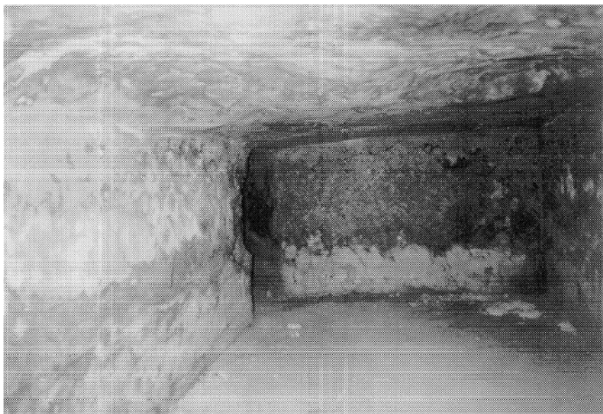
Figure 15.6. View into west tunnel from Asklepion, Corinth. The regularity of this tunnel indicates its construction or enlargement by man, but given the karst features of the geology here, this tunnel in its original form is likely to have been carved by flowing water. This so-called reservoir is 2.5 meters wide.
