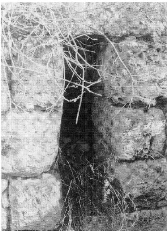
Figure 12.2. Slit in ramparts near the postern below the House of the Official, Morgantina. Such slits permitted runoff from inside the city to escape, possibly into an irrigation system outside, rather than build up behind the walls and endanger their stability. The slit is too small for anyone but a small child to penetrate, being approximately .3 by .6 meters.
