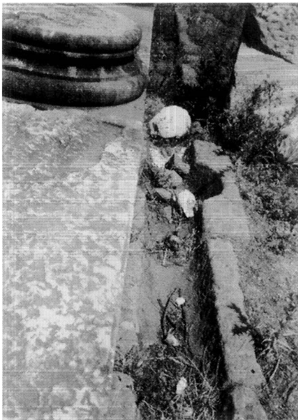
Figure 22.1. Eaves gutter and settling basin, gymnasium, Pergamon. The gutter is approximately 25 centimeters interior width.
