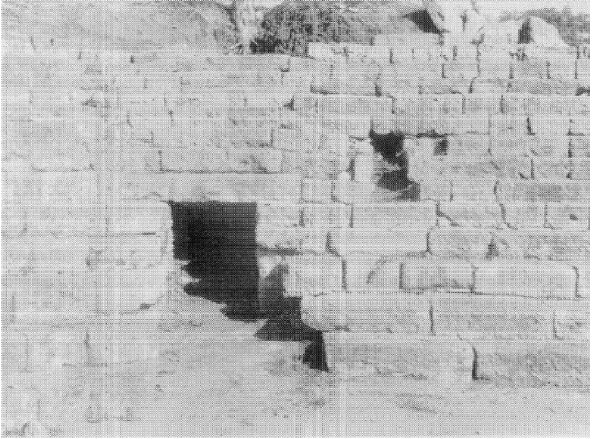
Figure 14.3. Large drains at two levels, piercing the Great Steps in the Agora, Morgantina. The higher one to the right seems to have become necessary after the lower part of the steps had silted up. The larger opening is nearly a meter wide.
